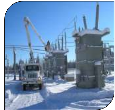
Missoula, Montana; FR3 fluid retrofill completed at -25°C.
